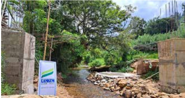
Restoration of Bridge in Varaniyawatta village
