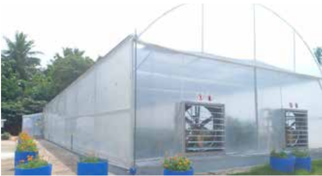
Fully automated Poly tunnel at Pannala
